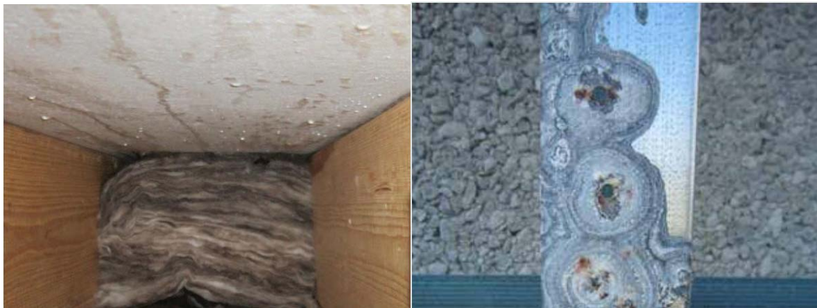
Figure 2-1-Evidence of damages due to MgO boards: Leachate visible on MgO board due to excessive moisture absorption (left) and corrosion of contacting metal framework (right) Source: (Hansen et al. 2016)
